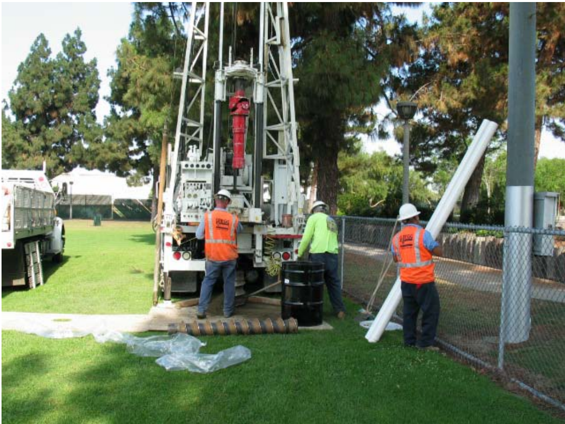
GMW-65 Well Installation
