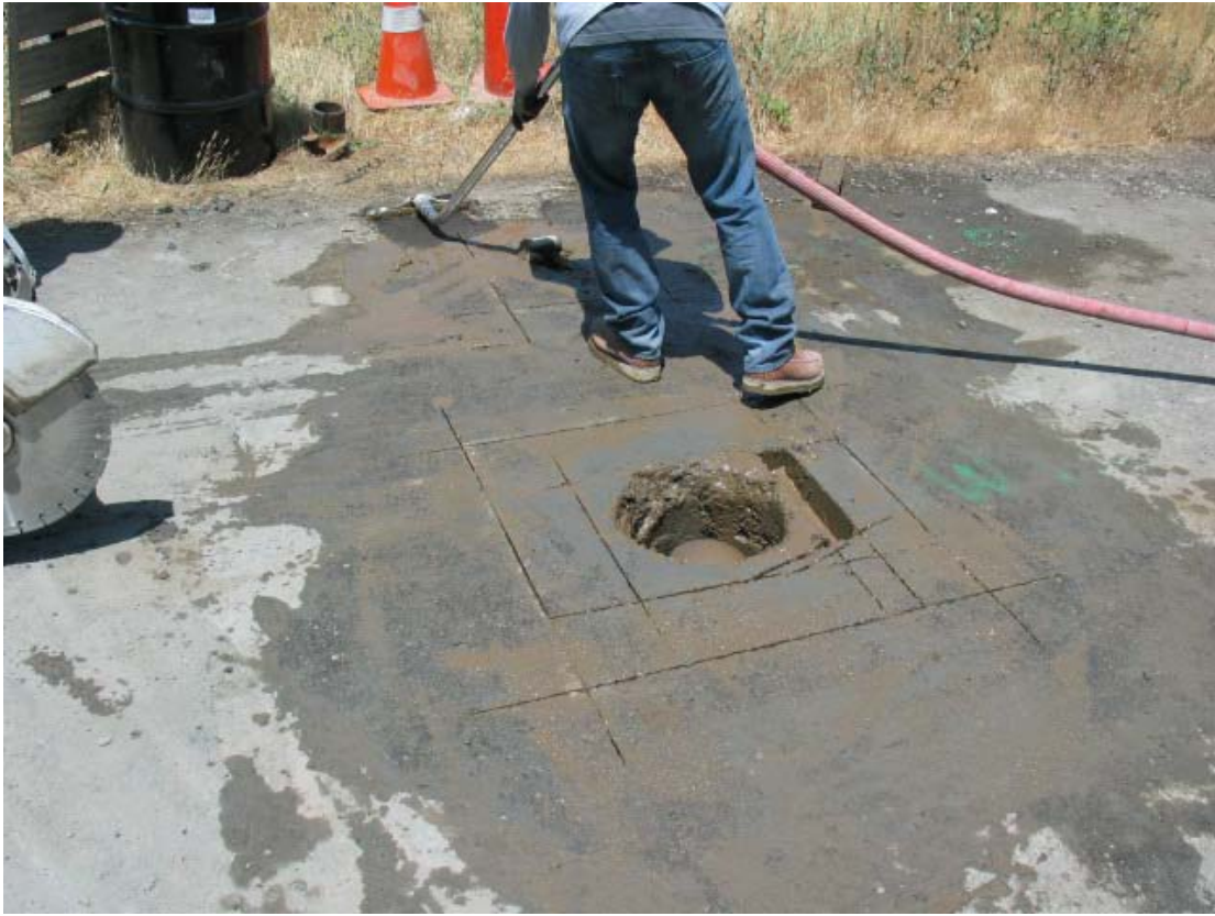
GW-16 Asphalt Cutting
