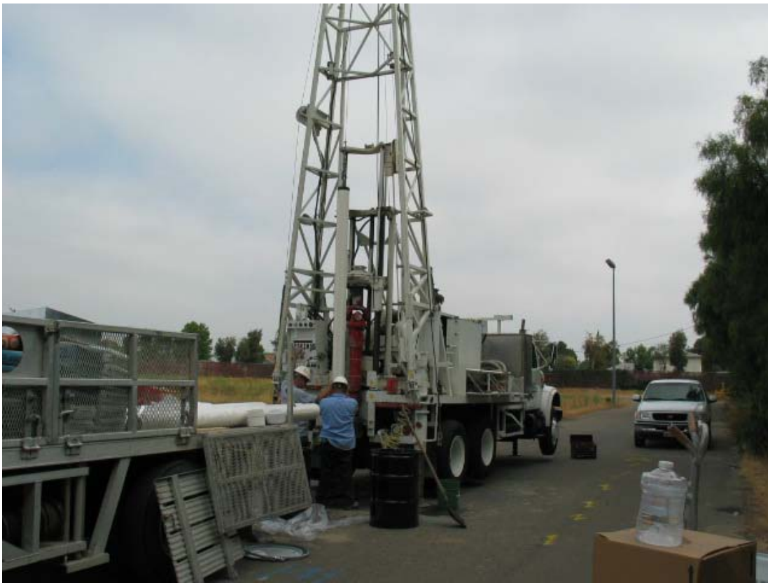
GW-16 Well Installation
